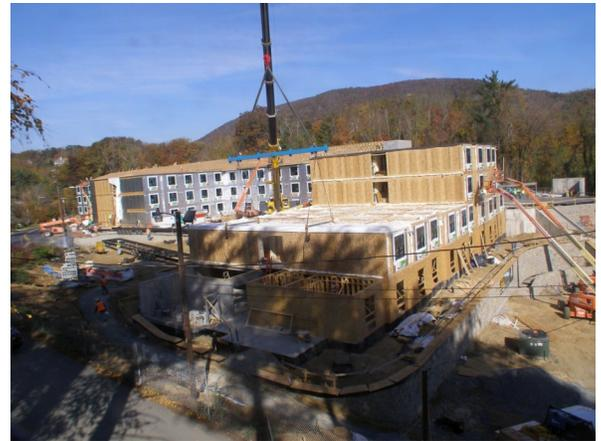
Hunter Modular Construction completed the erection of 129 modular units to form the 97,000 plus square feet permanent Residence Hall for ASU. HMC was contracted by Clayton and worked with JS Clark.
